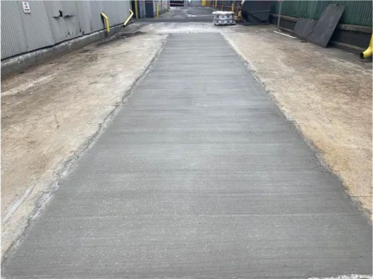
Image Description: Concrete slab repairs after fixing underground water line.
