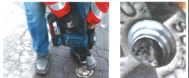
Figure 20. Drill hole and recess in chamber lid
